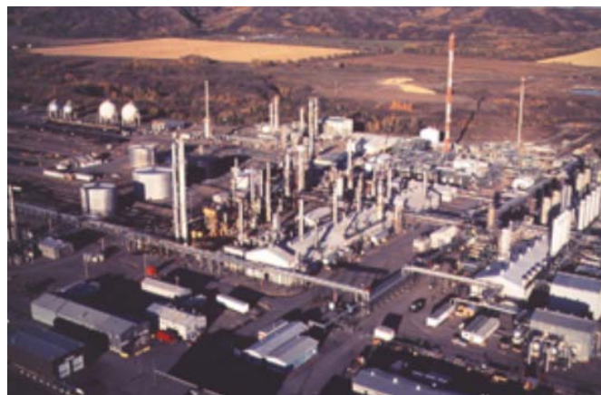
Figure 6- Gas refinery for producing natural gas product.
