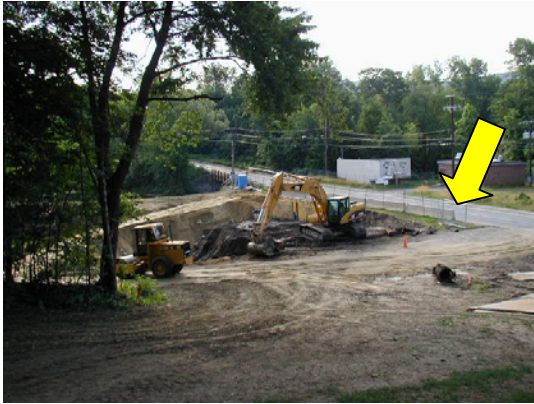
Figure 18- Downwind location (arrow) near active excavation of contaminated soil.
