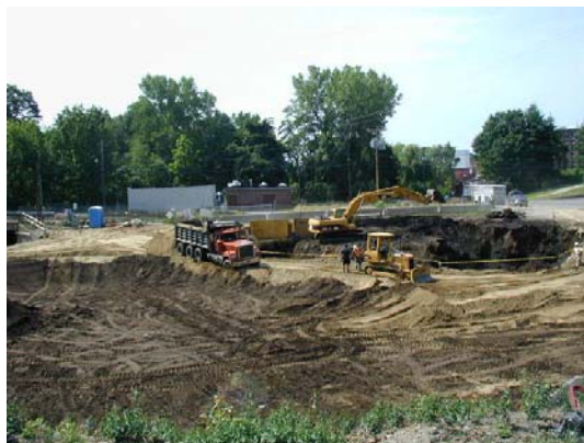
Figure 1- Excavation at remediation site involves removal of coal tar contaminated soil
